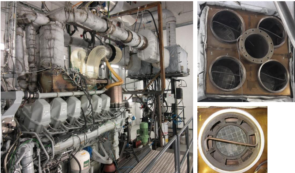
Figure 11.8.2 SCR coated DPF installed on high speed marine distillate R&D test engine, Frederikshavn
