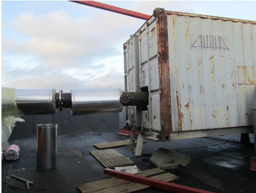
Figure11.7.2 Container and inlet pipe during installation
